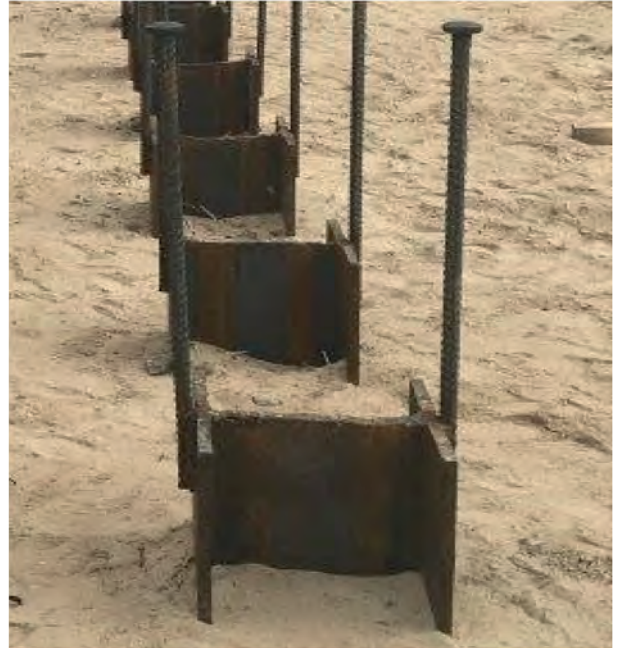
Welded Pile Anchorage
