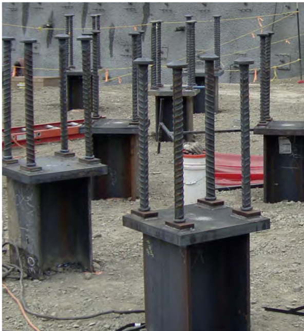
Pile Anchorage (w/ head plate)
