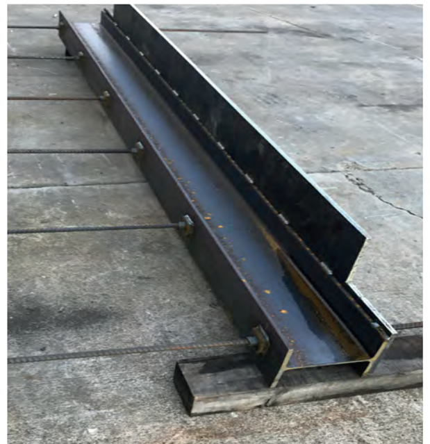
Dowels at Steel Beam/Lintel
